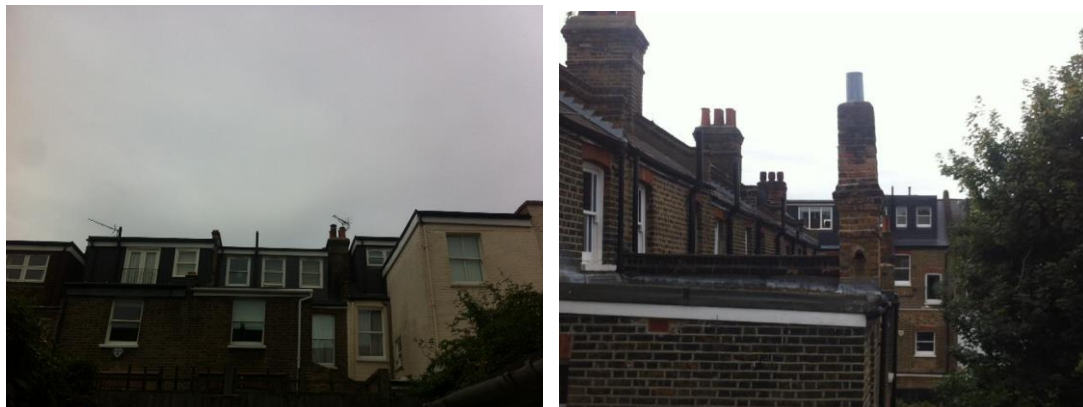
Photos 5 & 6 Existing dormers Calabria Road & Opposite along Liberia Road
