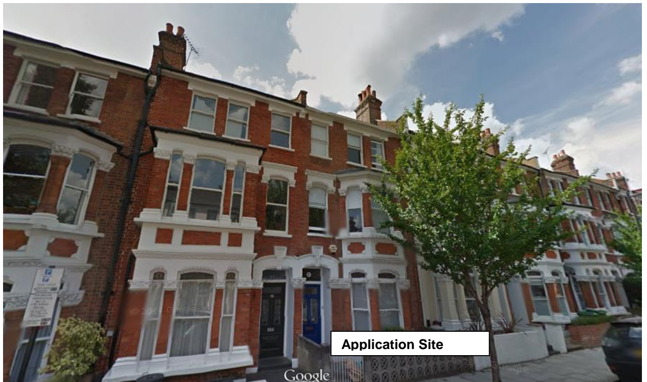
Photo 3: Existing front elevations along Calabria Road
